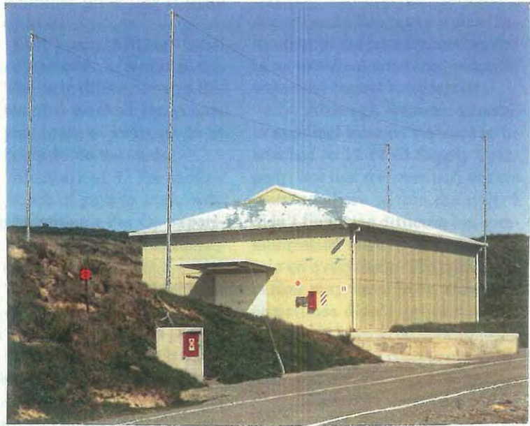
One of the refurbished buildings, complete with ramps, sealed road, and lightning conductors.
